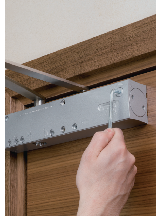
Door closer maintenance
